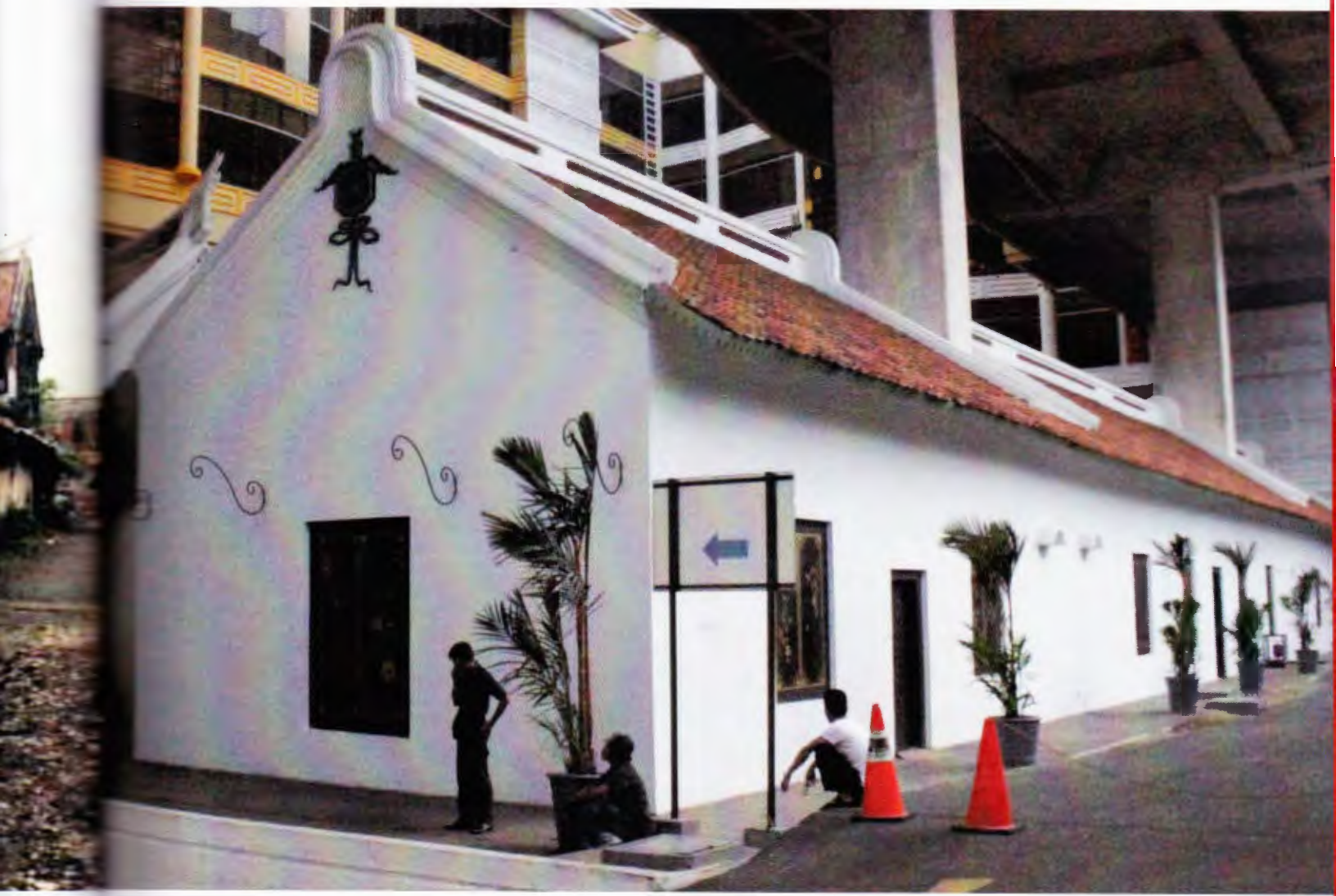
Kondisi bangunan bagian samping utara setelah dibangun kembali (tahun 2013) Building condition of northern side part after it was re-built (year 2013)
